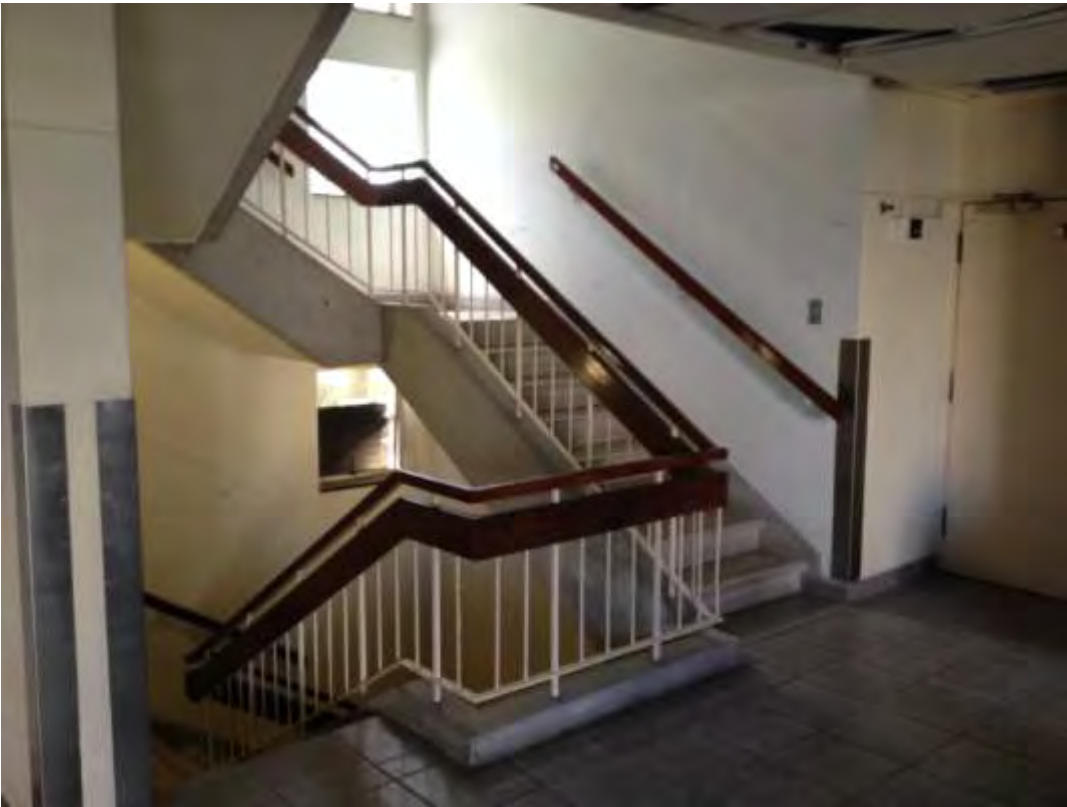
Much of the detailing is mainstream commercial modernism
