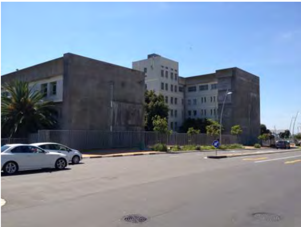
Three and 5 storey concrete-framed monolithic structures with repetitive elements typical of the 1960's and favoured for institutional buildings but not an outstanding example of modernist architecture.
