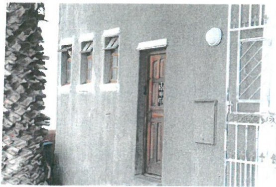
Doorway and bathroom windows adjacent to entrance
