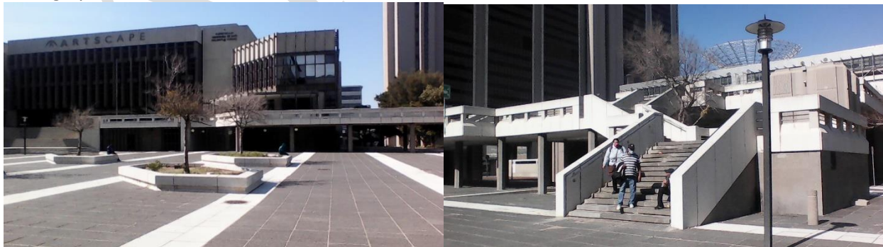
Figures 1 & 2: The Artscape Plaza/Forecourt with the main Opera House and steps leading towards the concourse.
