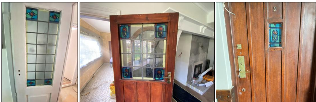
Figure 2. Various internal doors being used on site. The left door is the unapproved door, the middle door is a door being used elsewhere on the subject property, and the right door is the main entrance door for the subject property. Note that these similar but distinct typologies, as discussed above, are considered compatible for use on site from a heritage point of view.
